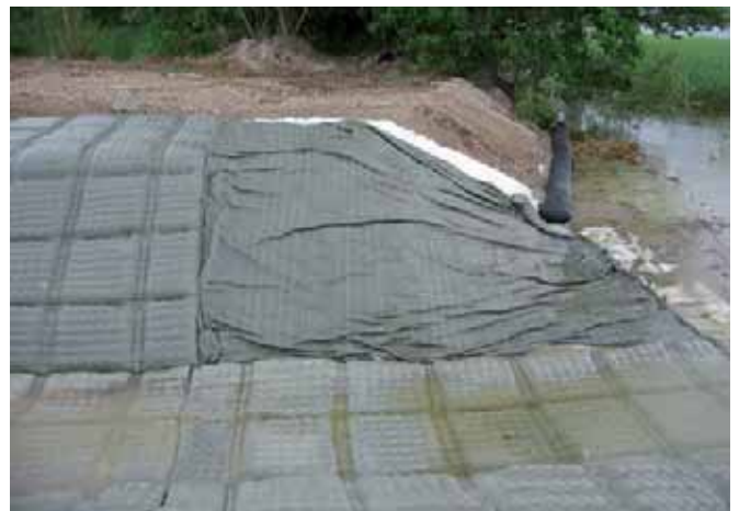
Pose (sections remplies et non remplies) (3)
